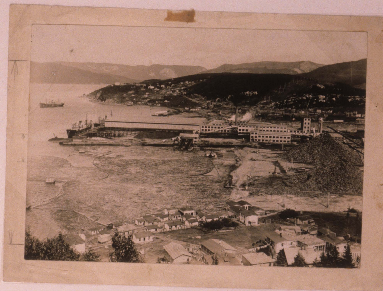
THIS AERIAL PHOTOGRAPH OF THE PAPER MILL AT CORNER BROOK WAS USED TO PREPARE THE VIGNETTE FOR THE 8¢ STAMP. THE AREA TO BE UTILIZED AND THE REDUCTION TO STAMP SIZE IS SHOWN IN THE LEFT MARGIN.
